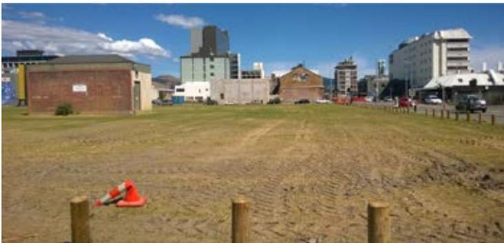
*Leveled, cultivated with hydromulch and seed on top. Germination is critical for dust suppression as well as ground stability. (photo taken 18/2/14)*
